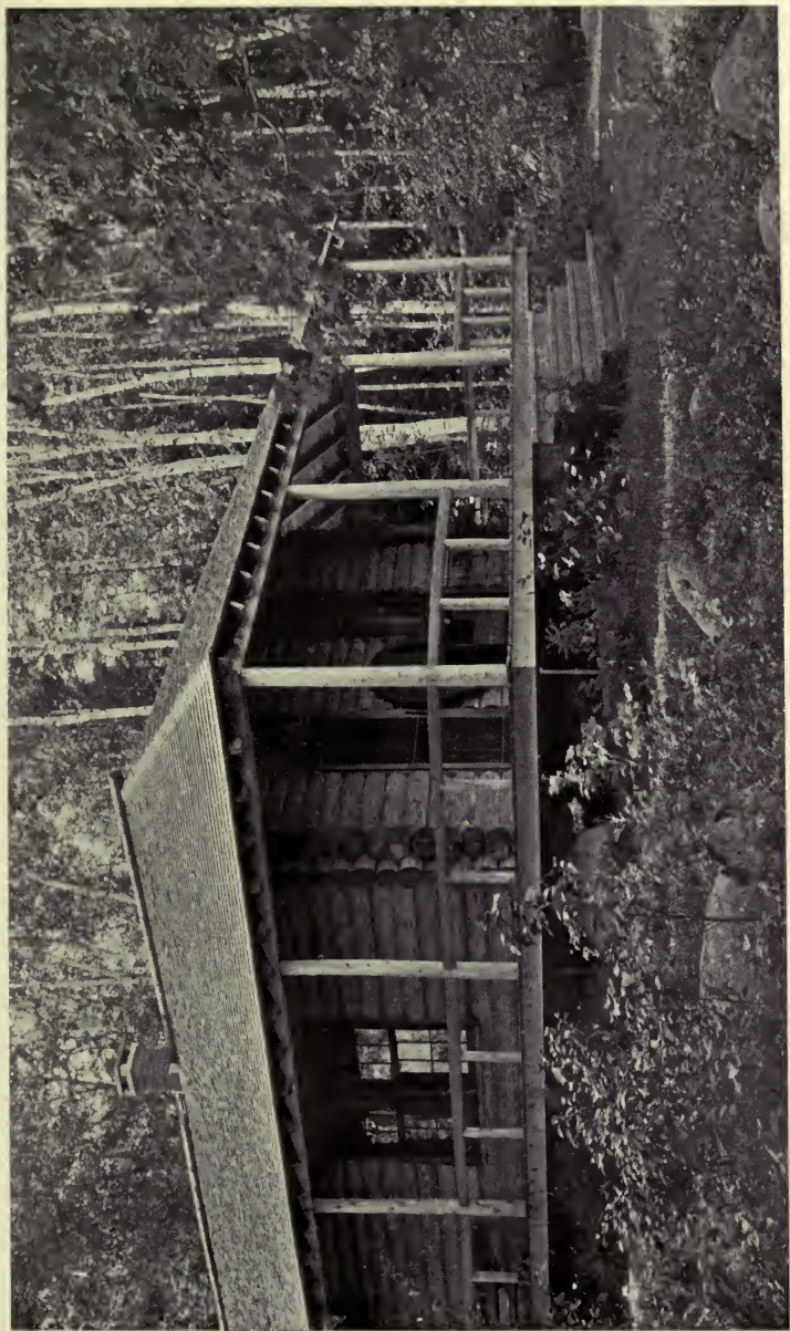
The Saddle-board is of Peeled Logs Fitted in Position. Note the Tall Windows in the End which are Hinged and Also do Duty as Doors. The Porch is Supported by Slender Iron Rods. In very Cold Climates this is Desirable, as the Frost Cannot Get Sufficient Purchase on the Rods to Heave the Structure.
