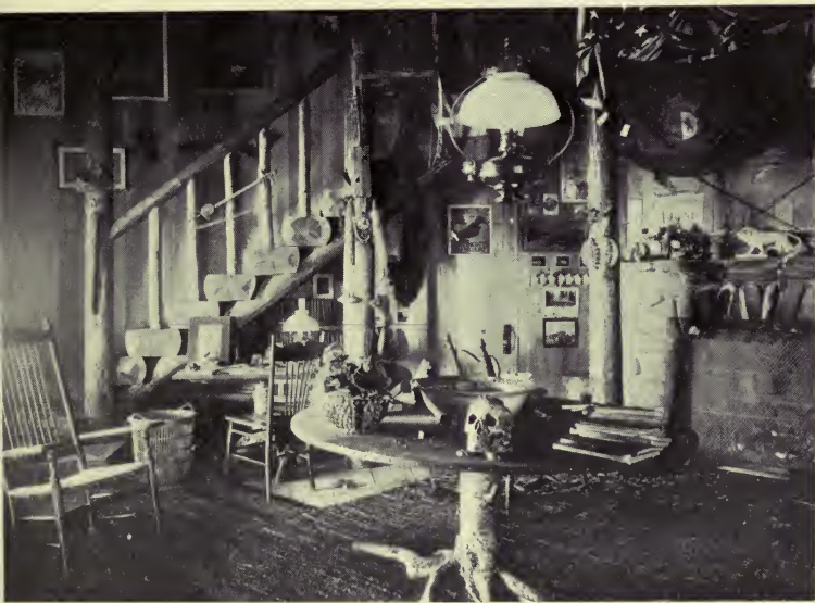
An Interesting Stairway. The Treads are of Solid Norway Logs.
