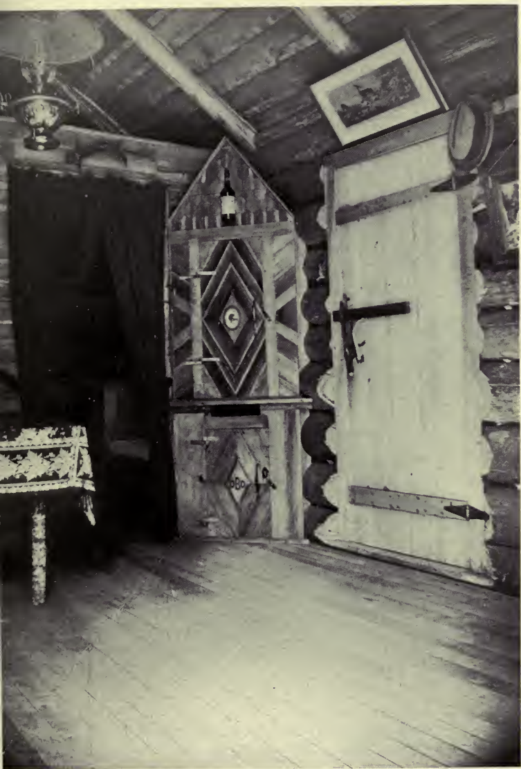
A Unique Closet for the Camp. Note the Beveling of the Logs Around the Door.
