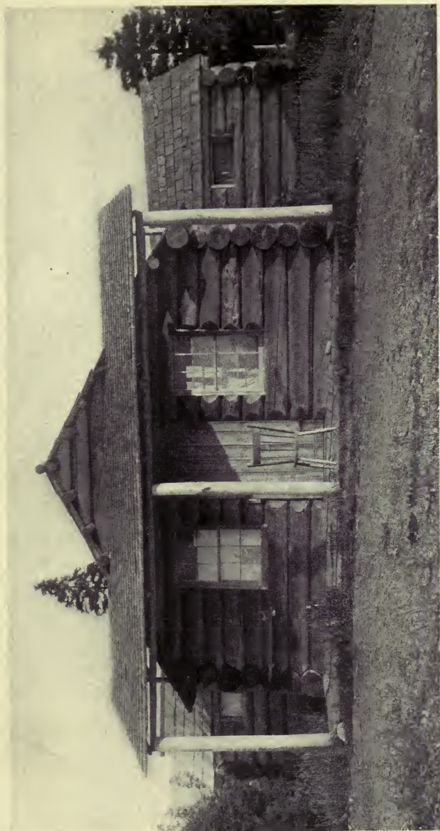
Note the Beveling of the Logs Around the Windows and Doors. Shows the Method of Setting in Rafters when Run Lengthwise of the Cabin.
