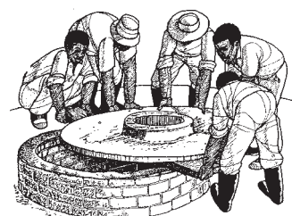
Set the cured well cover in place
