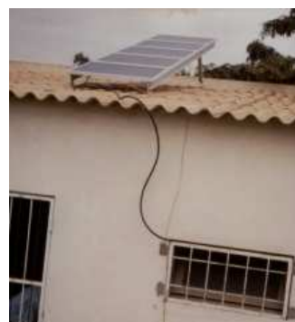
figure 30: mounted array
