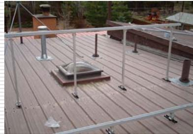
Although installation could be done by one individual, a multi-crew installation makes holding the rails to the vertical supports much easier. These rails are aluminum and easy to cut and hold in place.
