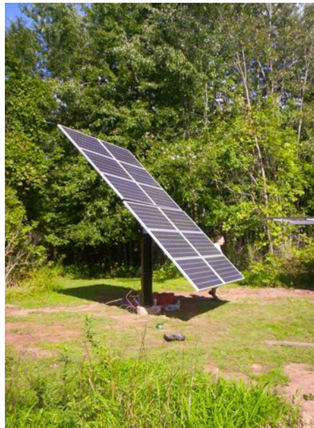
A ground mounted system, also called a 'pole mount' (running child not included).
