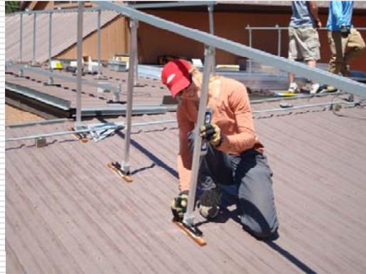
The installer works to keep the legs and rails plumb. Care is given during the "setup" stage to prevent having to disassemble or make major adjustments once the panels are installed. This system has a total of 33 Sharp 170 watt panels or a maximum production of 5.61 Kwh. The layout and rack installation took 2-1/2 days to complete (prior to installing any panels).
