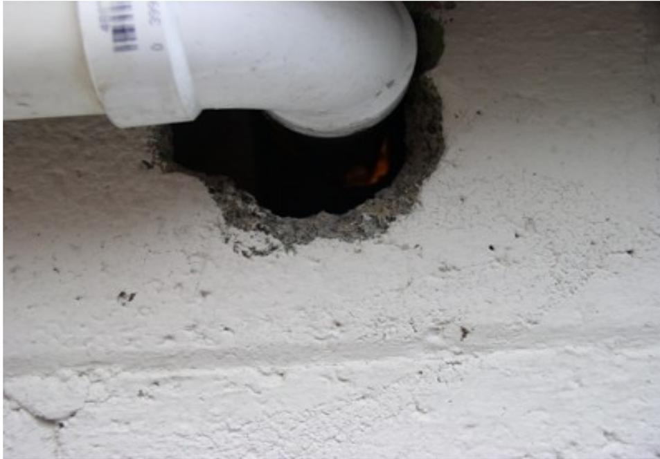
Check out this closeup of a gap between a sump pump pipe from a basement to the outdoors. Believe it or not, that “orange glow” is actually the lights inside the basement! Amazingly, the homeowner had no idea this problem even existed – until he did an energy audit...five years after he bought the house!
