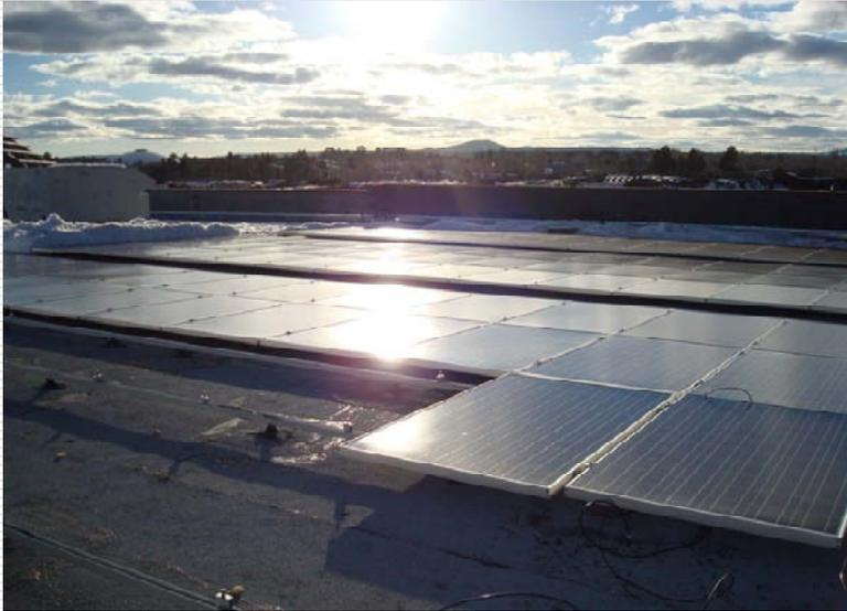
The racking system for this installation is laid flat on the built up roofing system. Care must be taken to interconnect the panels before they are lowered and connected. Obviously, maintenance to an interior panel is more complex.
