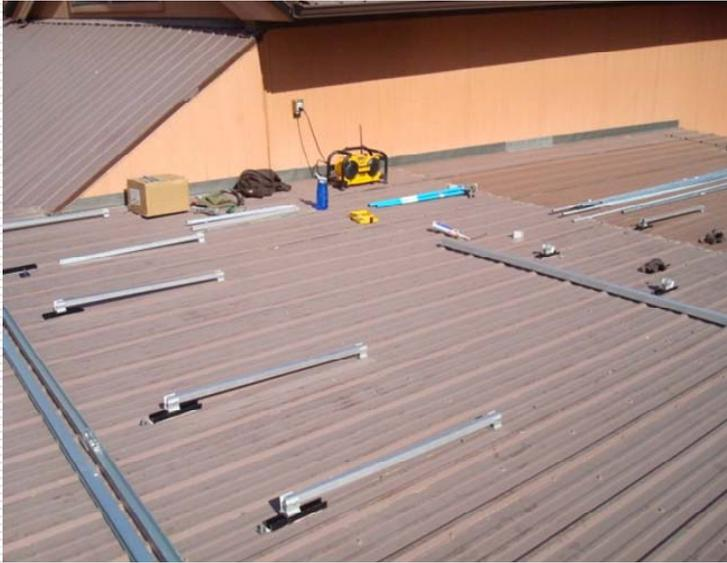
The front "rails" will have small restraining clips to hold the front of each panel. The vertical uprights [shown behind the rail] will elevate the panel to the desired angle for the specific latitude of the project. The clips are adjustable from side-to-side. For the vertical support legs (once cut to the correct length) also allow the installer to adjust the tilt of the legs. This system will be set @ 35 degrees (optimal for Flagstaff)
