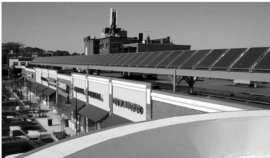
**This 20-kilowatt PV system produces electricity for the common areas of a shopping center in Cambridge, Massachusetts.**
