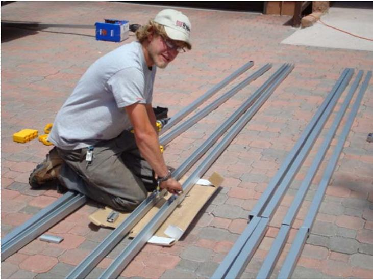
The alum. "C" channel shaped rails are connected together and must have a grounding bond between the rails. Charlie is securing a pre-drilled connector that will snugly clamp two twenty foot sections together. A bonding scrap, using a lock washer straddles the two channels and is tightened down. The Weeb splicers are used as the grounding is not sufficient with just the ProSolar splice kit.
