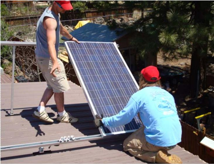
The first panel goes in and the installers check the racks for plumb and alignment. There will be a total of eleven (11) panels per array. The Sharp 170 watt panel being used here is guaranteed for 25 years. The open current voltage is 43.2 volts, the Max power is 34.8 volts, the Max current is 4.9 amps and the model efficiency is 13.1%. The panels weigh 37.8 pounds each and are 62"x32-1/2"x1-3/4" in size. (array configuration depends upon the maximum size of 600 Volts, DC)
