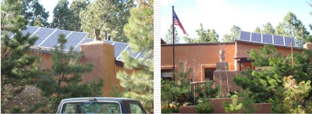
From the street side, this roof top solar panel generating system (5.61 Kwh) awaits the City inspection and "green tag". Once that it completed, APS is scheduled to replace the service panel meter with a bi-direction digital meter and approve the installation for operation. Then during the peak months, the owner hopes to run the meter backwards as it generates more than used.
