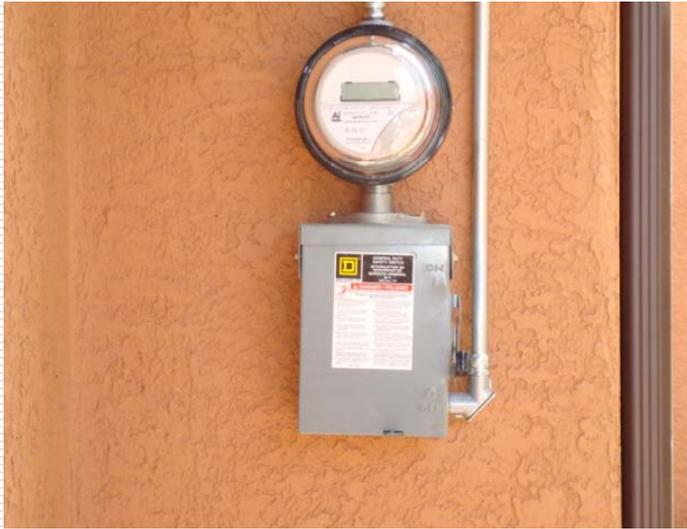
A digital AC “power” production meter is installed after the lock out junction box for the system. The Utility Company (APS) wants this lock out accessible without going into a fenced backyard. The meter must be read once a year and the information sent to the Utility Company within 15 days.
