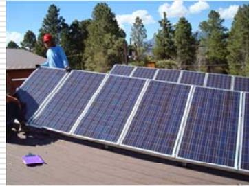
Panel arrays must be kept at the same angle (when the roof plane changes) to keep the voltage production the same. Some adjustments may be required; Kelly, Drew and Chuck are keeping the first panel square prior to tightening the lags.
