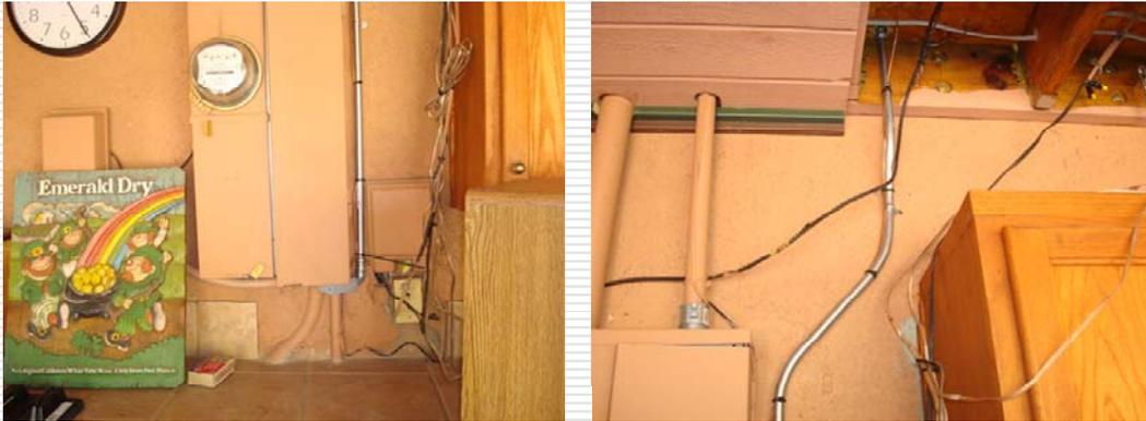
Since this panel is exterior to the house (open to the environment), the panel needs to be connected through the bottom of the existing service panel. The bare copper wire is connected to the service panel grounding lug and uses the existing UFER to complete the ground.
