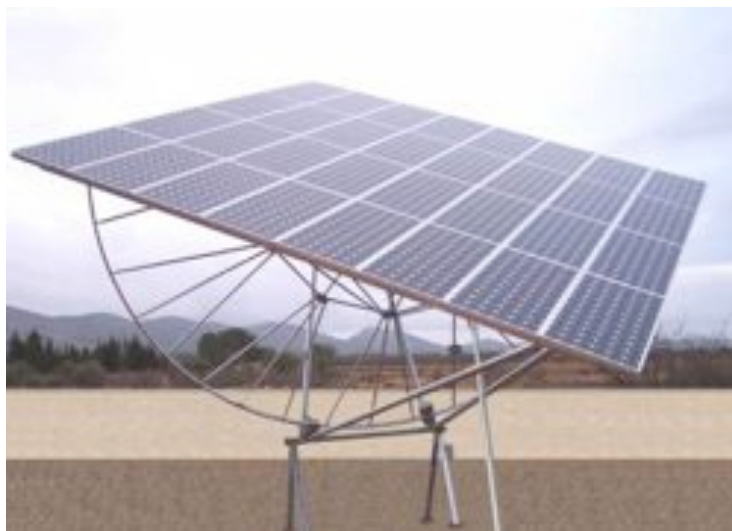
A dual axis tracking system, note the lack of shading and low horizons.
