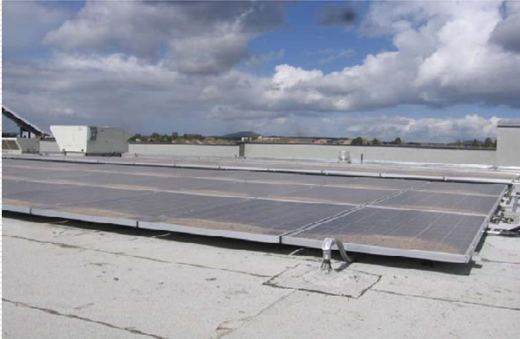
The electrical boxes (at ends of panel arrays) and conduit with conductors for the connections to the inverter bank(s) are snaked through a roof mounted and protected conduit (shown in the foreground).
