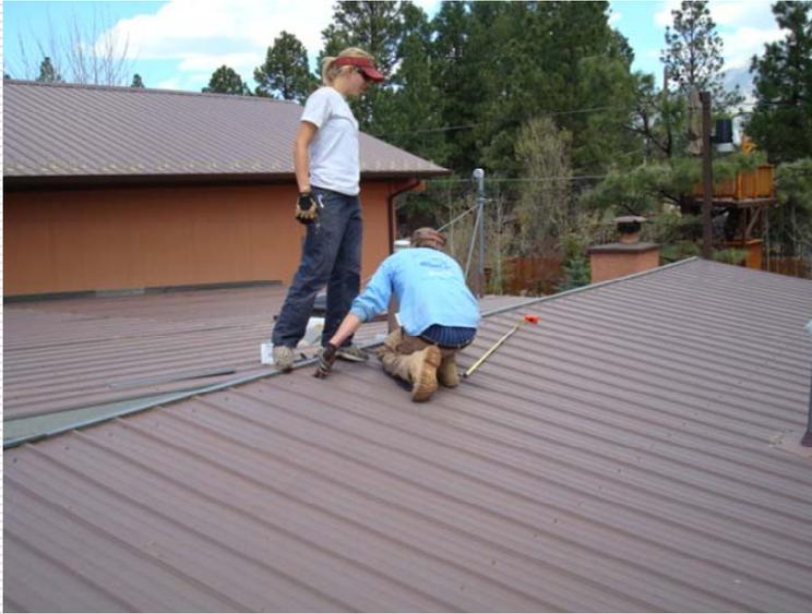
The layout crew will measure the surface area of the roof and must check the exact location of the roof framing members beneath. Since the panels add a tributary load of between 3-5 psf, this extra dead load is minimal and should not require a structural engineer. However, the rack system requires that the anchors are embedded into the roof framing, not just the sheathing.
