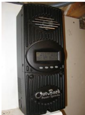
A 60 amp off grid charge controller
