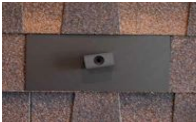
A Quickmount system with colored flashing. An attachment bolt is fed through the hole and into a rafter.
