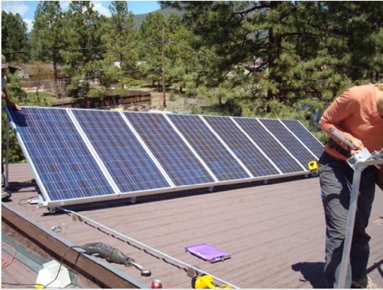
Typical roof top installation uses a rack mounting system, panels set in arrays or "strings" (multiple panels) and conduit for interconnection of panels. Shown here are Sharp 170s. A cell or module is a single silicon unit and generates 0.5 volts.
