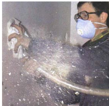
A contractor installing blown-in insulation, a nice way to add additional insulation to an existing home.
