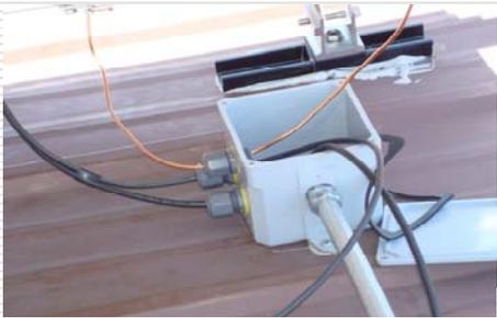
The proposed system would allow standard 12 gauge wiring; however, going to the next larger size (10 gauge) is more efficient and doesn't cause voltage loss to heat because the gauge is marginal or undersized. Because this is a metal roof installation, THWN 90 high heat wiring and insulation were used.
