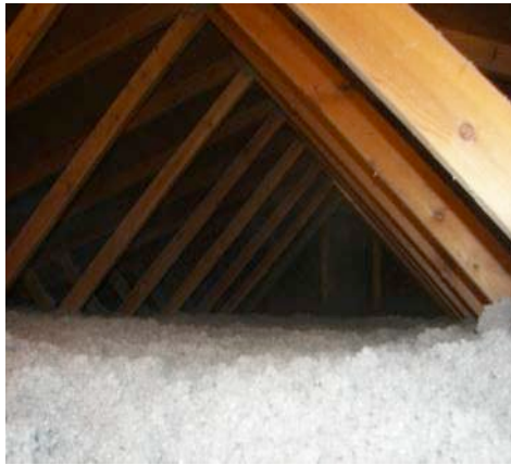
Blown-in insulation in an attic.
