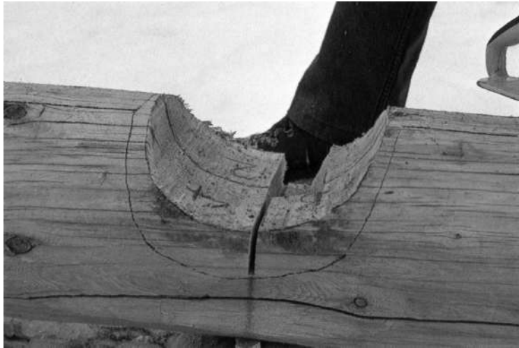
STEP 14: Quadrant #1 is removed by first cutting a small "v".
