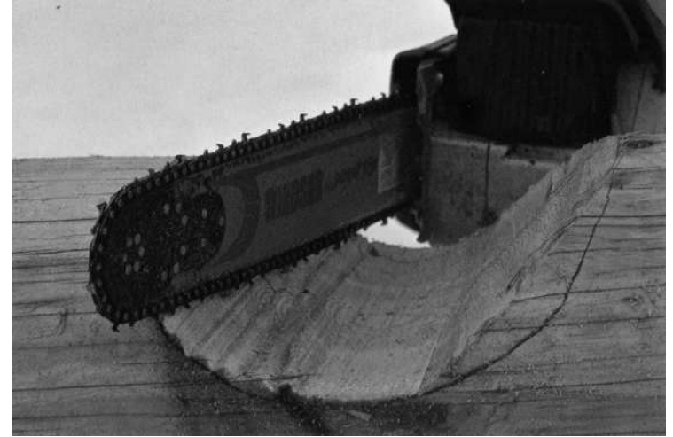
STEP 13: By crossing over the stepped cuts, the builder now smooths the notch.
