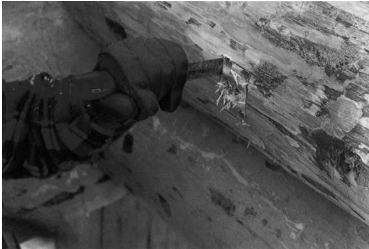
STEP 5: The rectangular hole may now be chiselled to accommodate the box.
