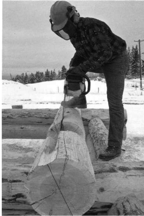
STEP 24: By rotating the log (note the 'Plumb Line'), and using the initial saw cut as a guide line, the lateral cut is made along the length of the log.
