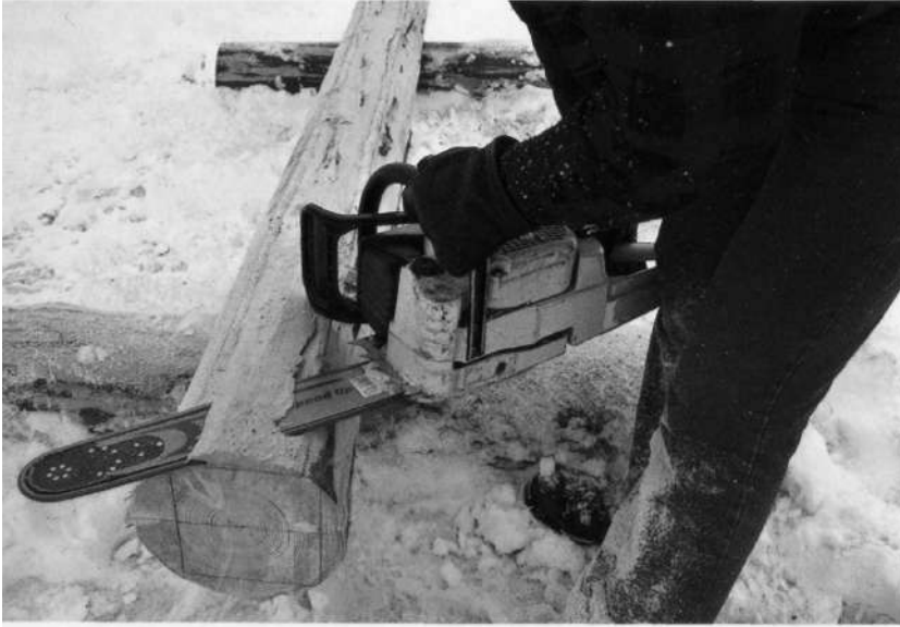
STEP 15: Correct procedure will guide the builder to the end of the log and very little touch-up work will be required.
