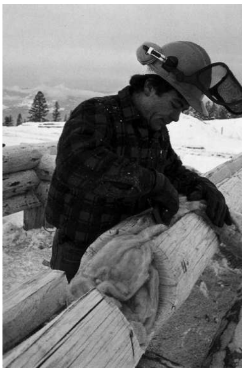
STEP 27: Once the log has been correctly fitted, insulation is stapled in the notch and along the lateral groove. (At the time of this publication, materials other than fibreglass are being experimented with and the reader may wish to choose an alternate insulating material).
