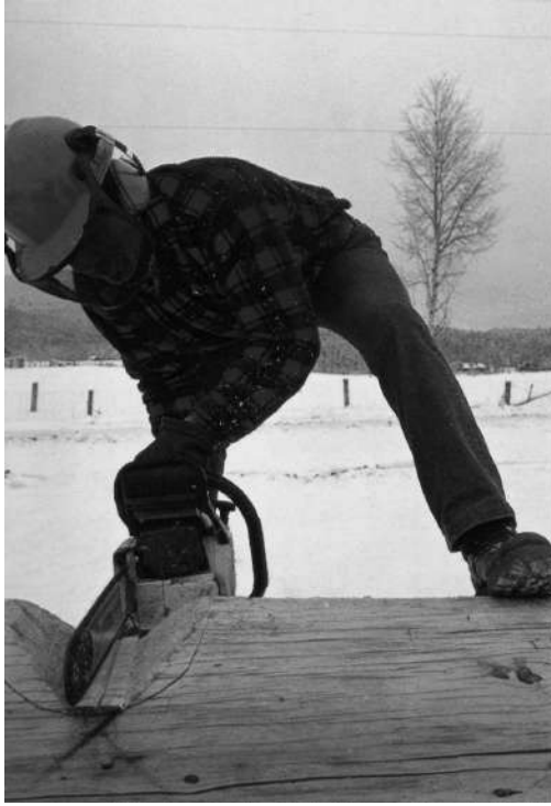
STEP 11: With an axe, remove the two wedge-shaped pieces of wood. Smooth the bottom of the notch with a 'brushing motion'. Note that the chainsaw bar crosses over the original cuts.
