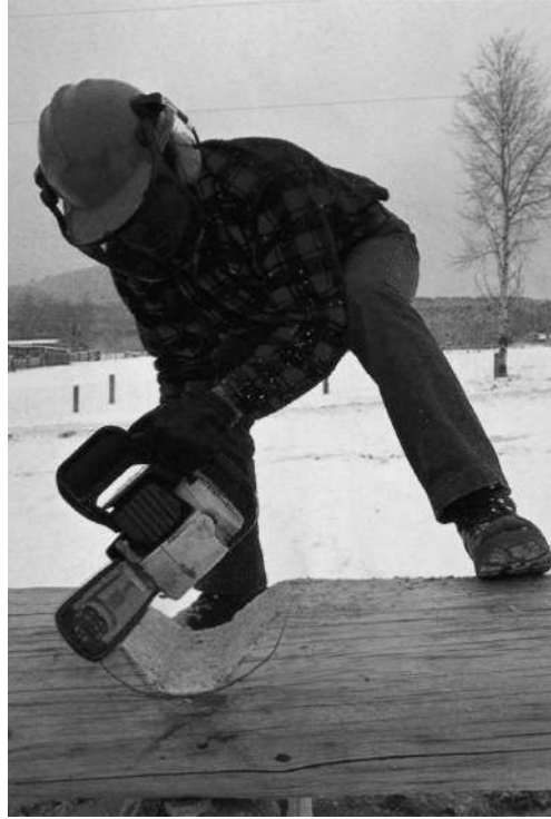
STEP 12: By using the full length of the chainsaw bar, a series of cuts are made, originating at or near the upper part of the notch, downward toward the centre. Note that the amount of wood removed by each cut is exactly the thickness of the saw kerf.
