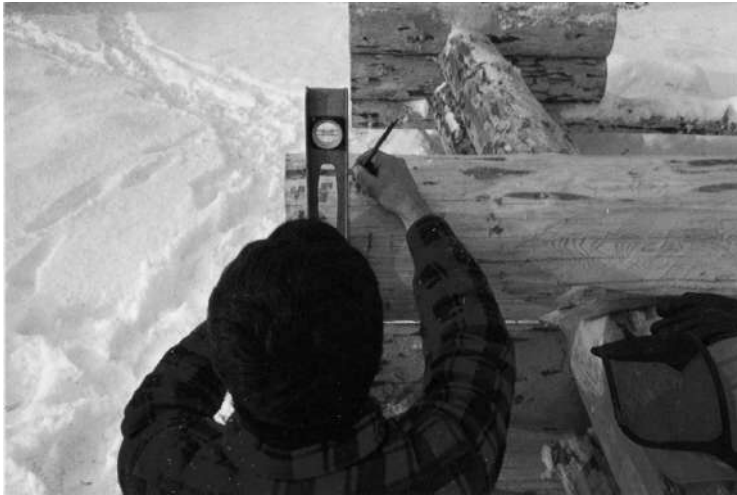
STEP 2: It's good practice to also sight to an opposing corner to get an accurate cutting line on the log.
