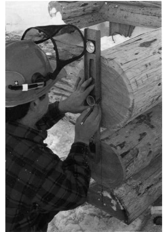
STEP 4: Once the ends are trimmed and the log is placed DIRECTLY above its final resting position, a 'Plumb Line' is put on the end of the log. By using the 'Plumb Line' on the preceding round as a guide, a line is placed on the working log with a level.
