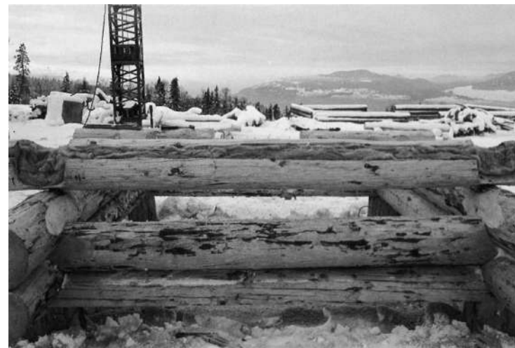
STEP 28: The entire log, from notch-to-notch, is insulated.
