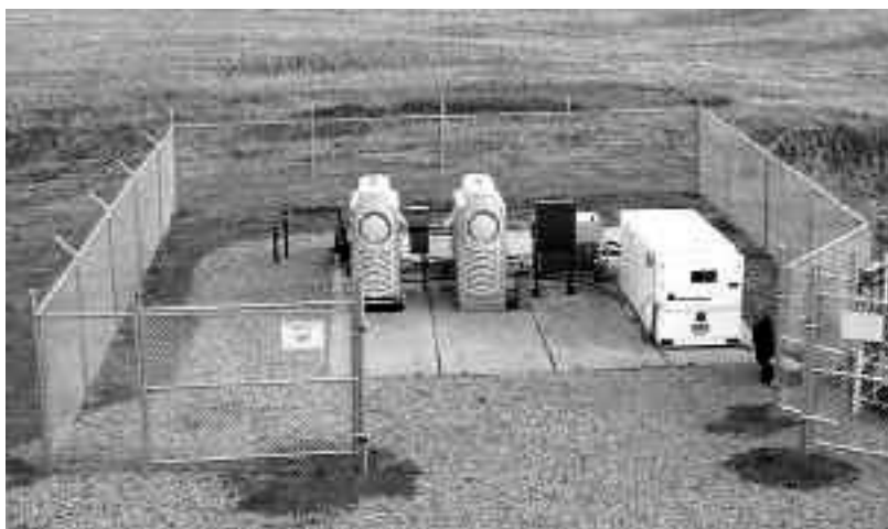
FIGURE 39.15 Aerial view of the PowerBlock® module with two microturbines near the Denver International Airport. (Source: From Reference 22.)
