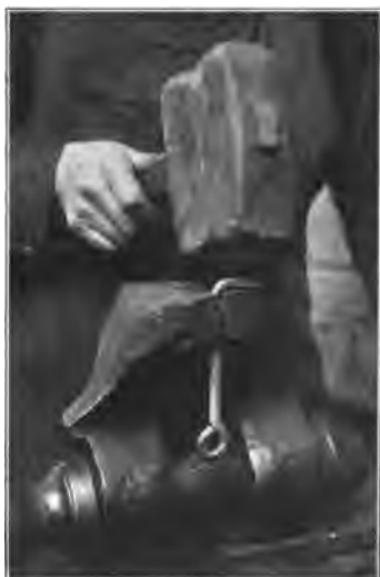
FIG. 17. BENDING HOOK IN THE VISE.
