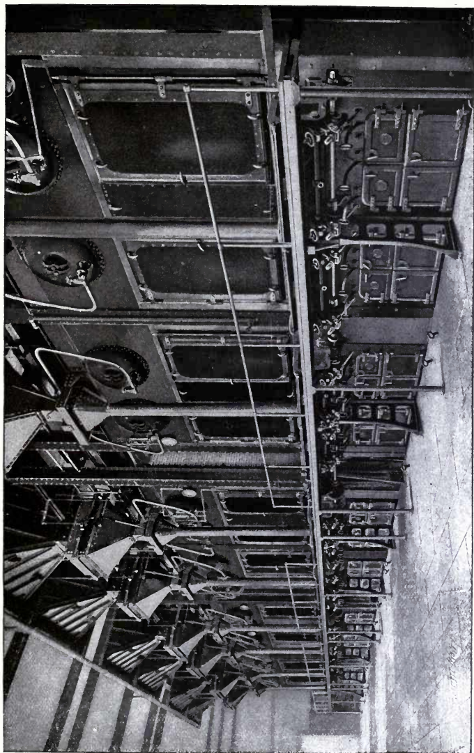
VIEW OF 4000 H. P. OF BOILERS AND RONEY STOKERS Installed in Plant of the Edison Illuminating Company, Boston, Mass.
