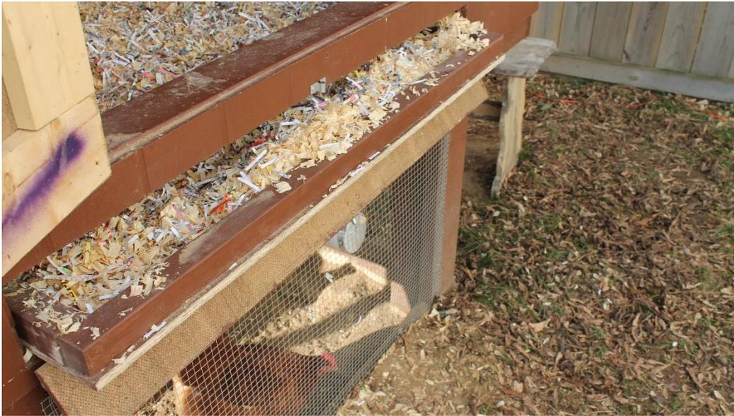
The cleanout tray is one of the best features of this design. The tray slides in and out along the floor of the coop through a small access door under the main access. The tray is made of scrap 2X4 cut into 1.5" strips and some OSB. I used deck stain to seal the wood and protect it and some cheap stick on linoleum tiles on the inside of the tray.
