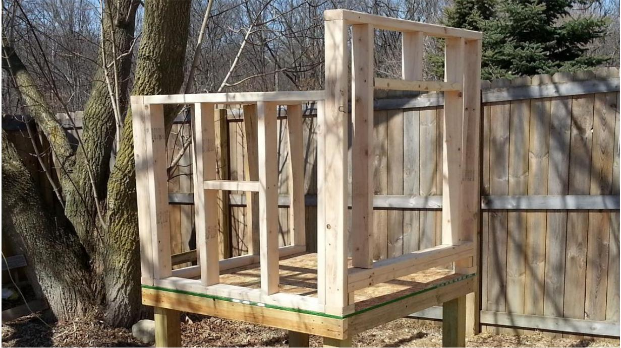
Each wall is constructed of 2X4 pine (most of which came from the 70% off bin at Home Depot). No wall is longer or higher than 4' to make efficient use of 8' 2X4's and sheeting. The front wall contains the entryway and cleanout tray access. The left side wall contains the chicken door entryway. The right side is where the nesting boxes will be attached.
