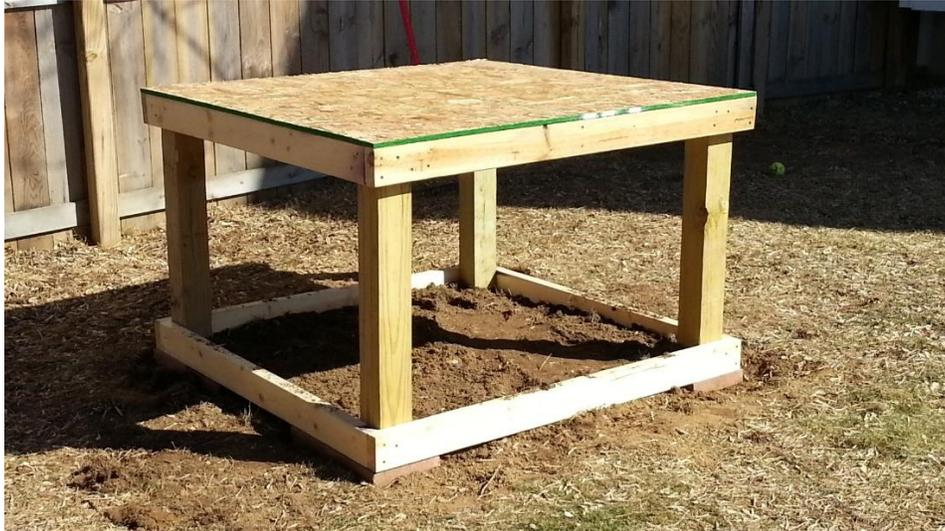
The first step is to level an area greater than 4' X4' to accommodate the base of the main coop. The base consists of 4 posts with a 2X4 frame to make it rigid. The outside diameter is no greater than 4' as to maximize use of 8' 2X4's. Each post is resting on its own pad made from cheap patio stones on level ground.
