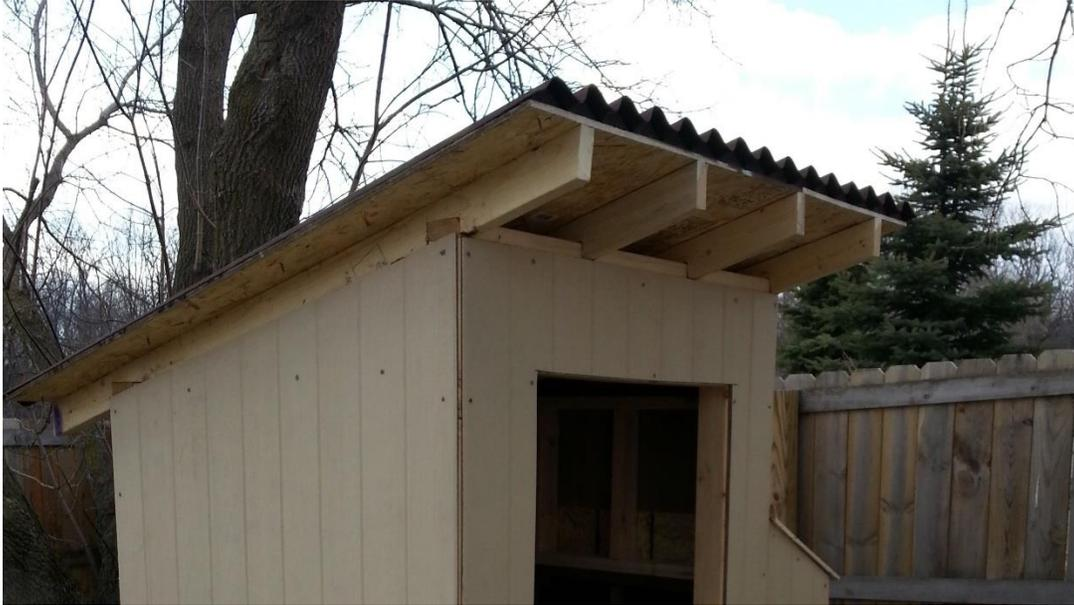
The roof is fairly simple, 4 2X4 trusses spanning from front to back. Each truss is notched out to rest on the front and back walls. The top is covered with OSB with as much over hang as you would like. The roofing is made of corrugated roof panels to fit over the OSB roof. There are special nails that go with the roofing panels and foam caps to close of the rigged ends as well.
