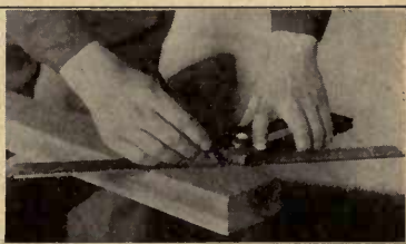
Fig. 80. Laying off Plumb Cut with Framing Tool
