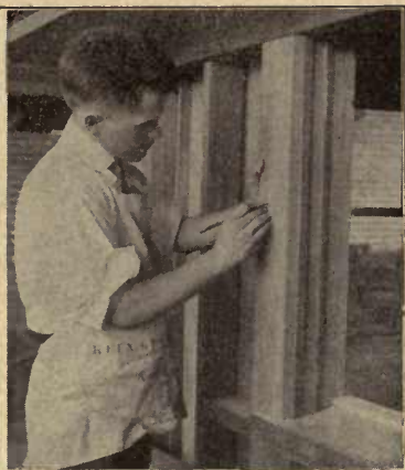
Fig. 113. Using Siding Stick
