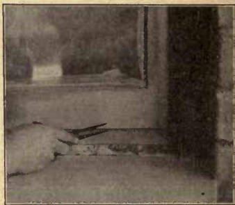
Fig. 130. Scribing Bottom of Lower Sash
