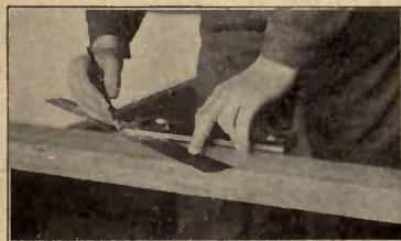
Fig. 79. Laying off Seat Cut with Framing Tool
