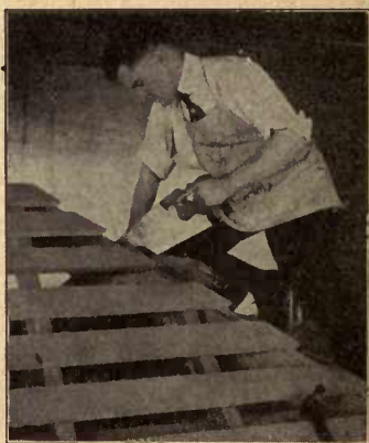
Fig. 92. Sawing Roof Boards
