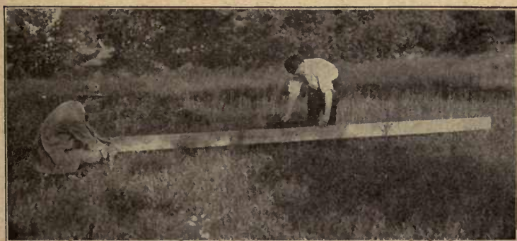
Fig. 6. Leveling with Straight-edge
