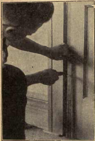
Fig. 135. Locating Hinge Position
