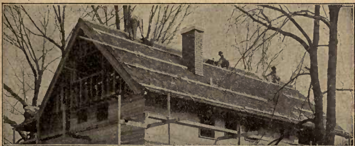
Fig. 104. Shingling. Toe Holds
