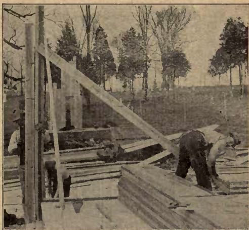
Fig. 33. Corner Post Being Plumbed and Stayed
