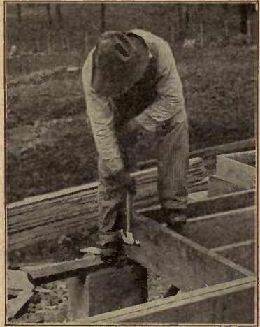
Fig. 26. Placing Headers and Trimmers
