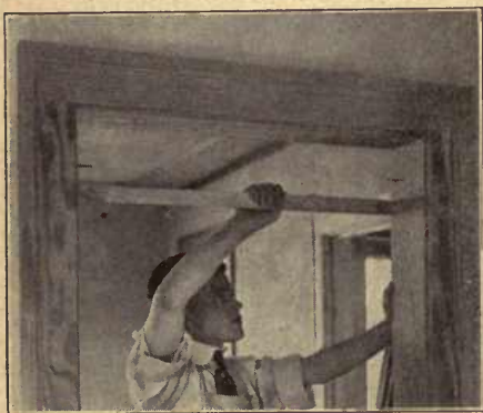
Fig. 133. Measuring Opening
