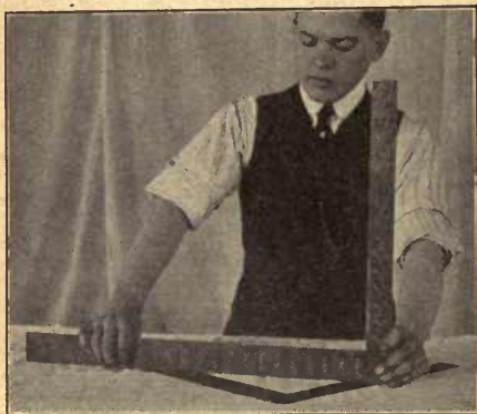
Fig. 51. Finding Rafter Length by Scaling
