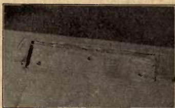
Fig. 139. Gain Ready for Hinge
