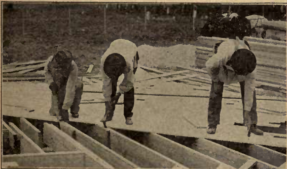
Fig. 27. Floor Frame and Rough Floor
