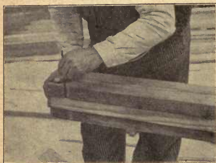
Fig. 31. Marking Joists from Pattern
