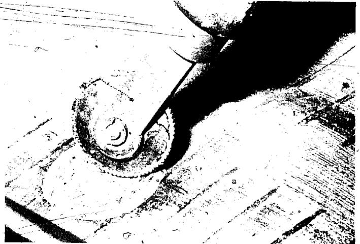
**STEP 14: Remove patch backing**, and center the patch on the hole using thumb pressure (right). **STEP 15: "Stitch" patch down**, working from the center to the edges. Then, remove the paper or plastic covering.
