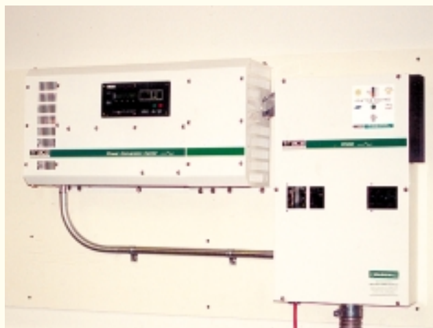
Trace 4 kW sine wave inverter and optional DC power center
