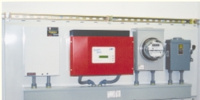
Sunny Boy grid-tie inverter, optional disconnects, and check meter
