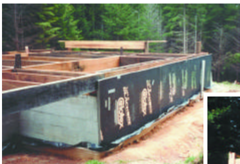
Above: The entire outside of the house is wrapped in an insulating envelope.
