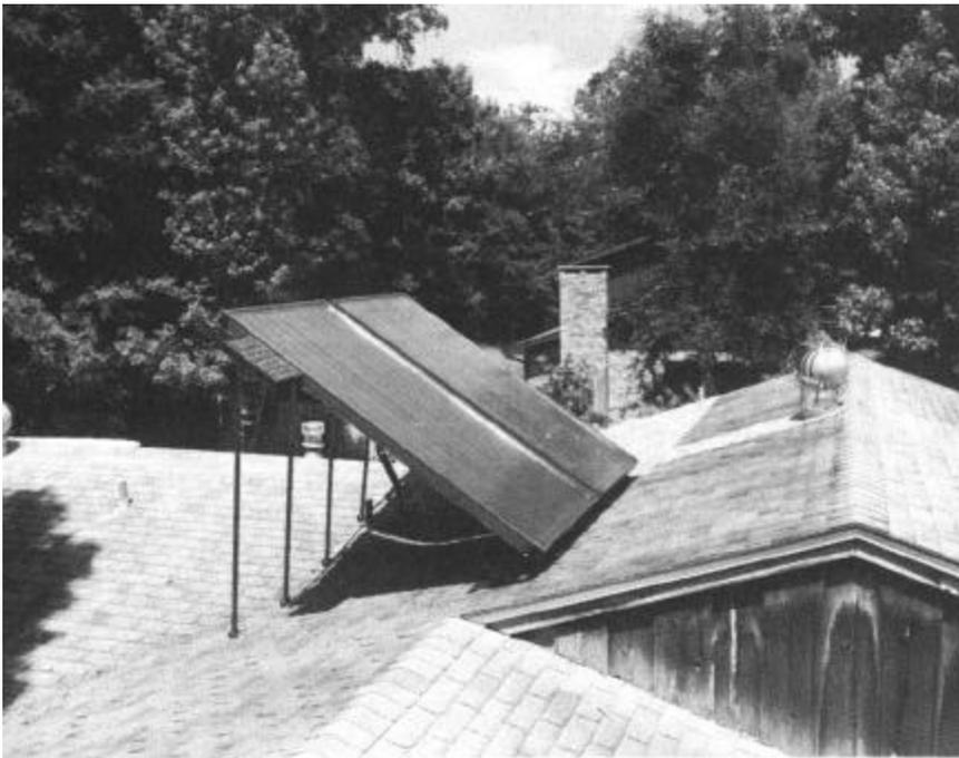
*Collectors mounted on the north roof facing south. This strategy keeps the collectors from being mounted on the front of the house. Note the photovoltaic panel attached to the side of the thermal panel.*
