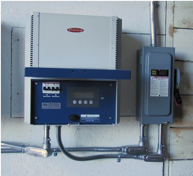
Photo 1: One of two Fronius 3-kW grid-tie inverters. Note the DC-rated safety disconnect and all high voltage wiring installed in metal conduit.
