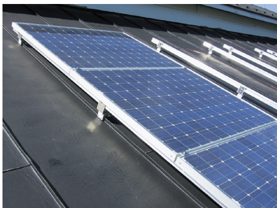
Photo 4: Start of installation of solar modules on raised mounting rails
