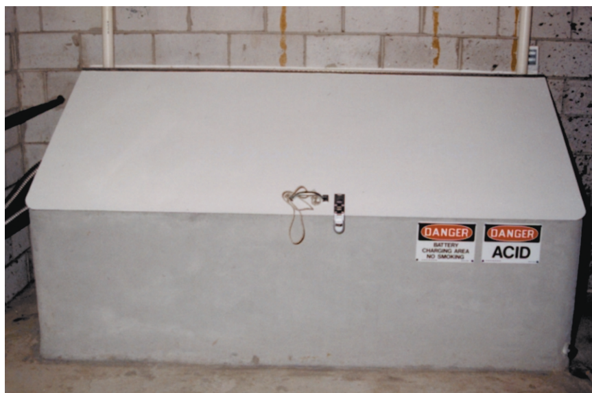
Air-tight insulated battery box with PVC air vents to the outside
