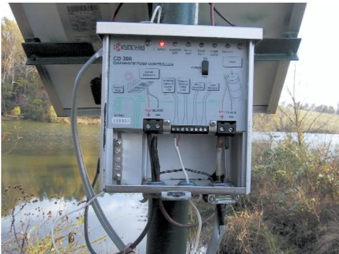
*Kyocera solar pump controller (cover removed)*
