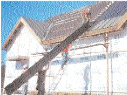
Left: A Uni-Solar module is lifted to the roof and installed.
