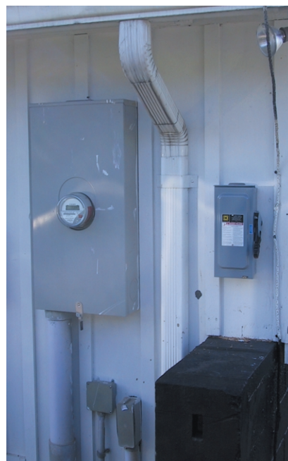
Photo 5: Utility required emergency solar disconnect located next to utility meter
