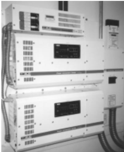
*Dual 4 kW Trace sine wave inverters to provide 120 and 240-volt AC power from a 48-volt DC battery bank*
