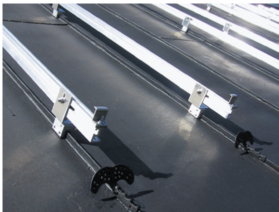
Photo 3: Solar array mounting rails and raised seam metal roof clamps
