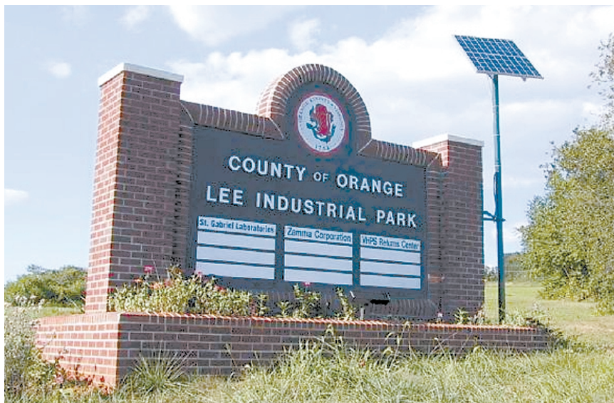
Figure 8. Solar powered street signage that includes: ground-mounted light fixtures located in the planter box on each side of the sign, a pole-mounted solar array mounted next to the sign, and a weather-proof box located behind the sign which contains the charge controller and 12-volt gel-cell battery.
