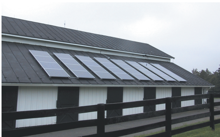
Photo 6: Completed solar array on south facing barn roof
