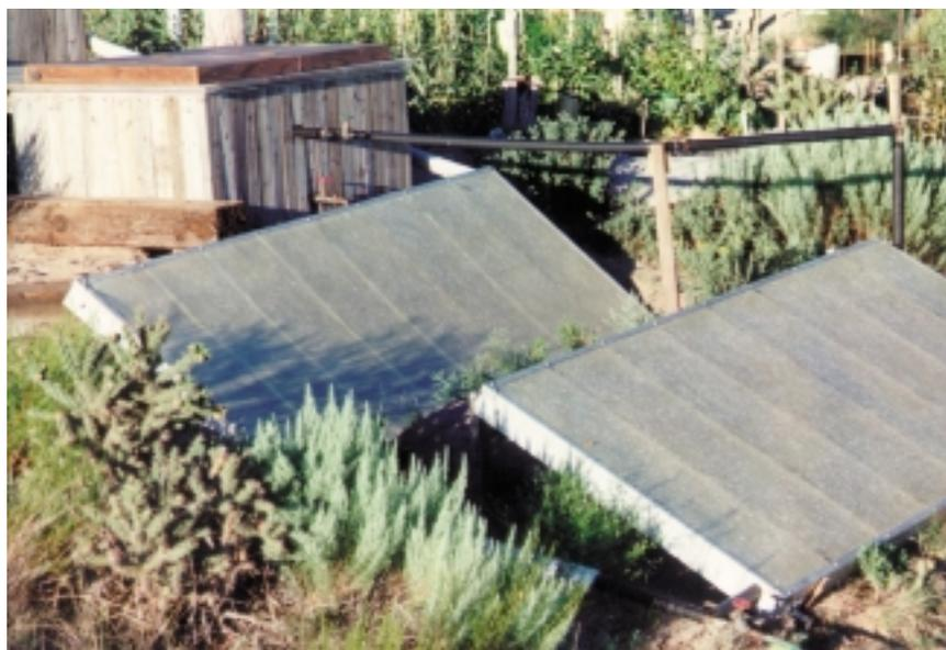
*Tub with collector (lower right). Upper collector is for domestic water heating.*
