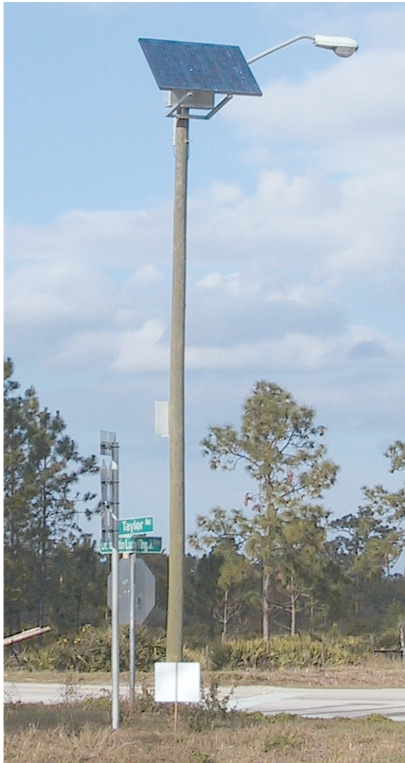
Figure 1. Pole-mounted street light showing a front view of the solar light
