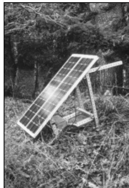
The original installation—two modules on a homemade cart to power a pump in the spring tank.
