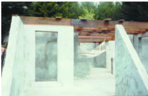
Left, above, & right: The foundation for the tower serves as structural and thermal mass and provides 300 square feet of comfortable living space.
