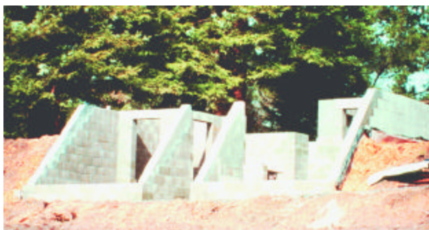
Left, above, & right: The foundation for the tower serves as structural and thermal mass and provides 300 square feet of comfortable living space.
