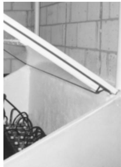
*Site-built insulated battery box. Note the gasketed lid and rear PVC pipe vent to outside.*
