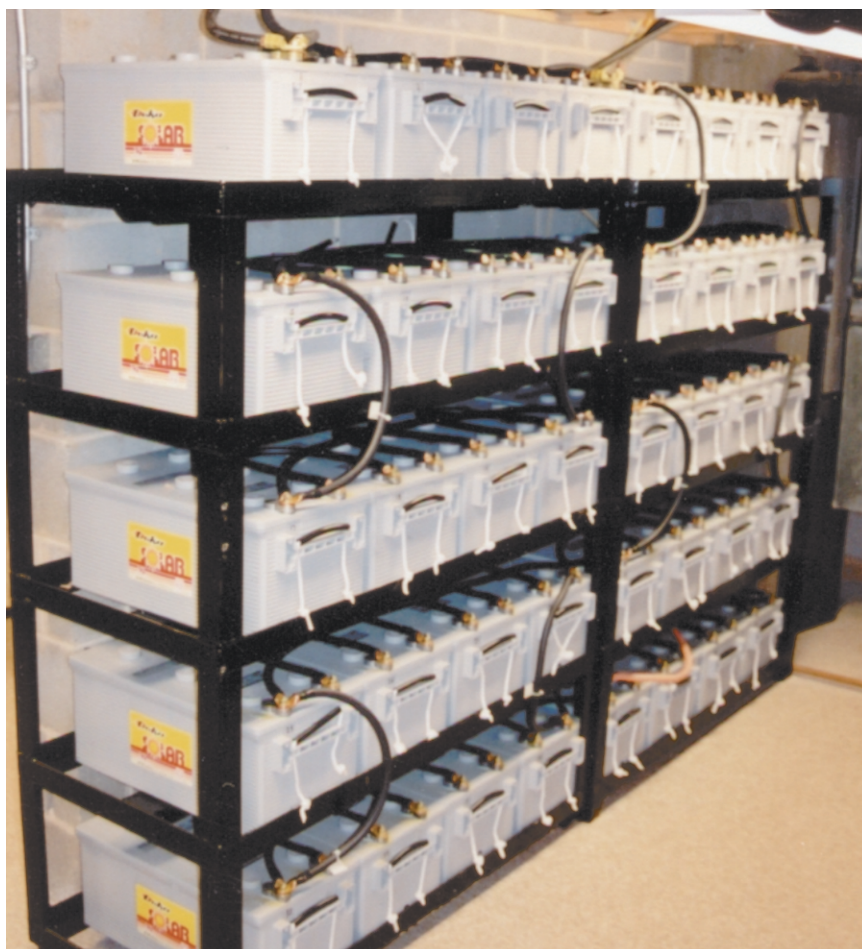
Rack-mounted solar gel-cell sealed batteries
