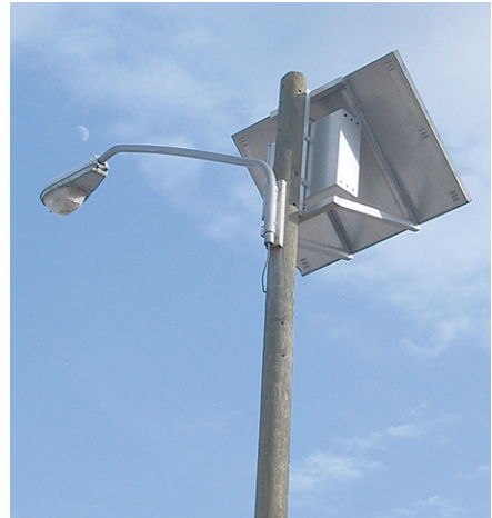
Figure 2. Rear view of a pole-mounted solar light
