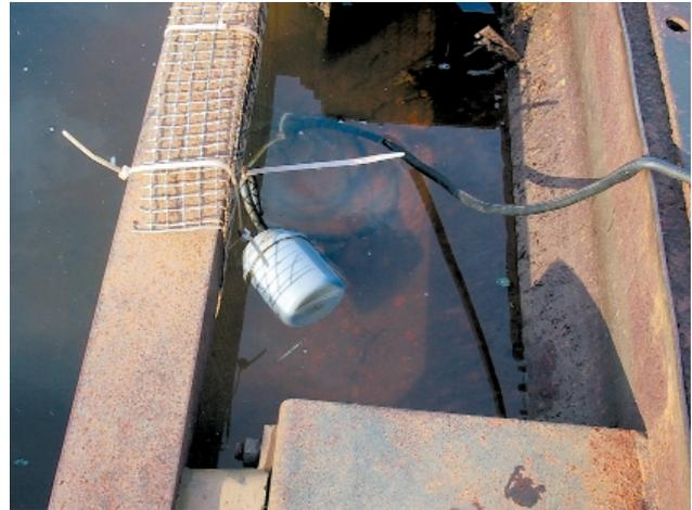
*Float switch in the tank to turn off the pump when tank is filled*
