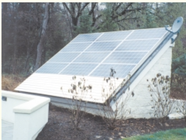
Kyocera solar modules mounted on outbuilding roof.
