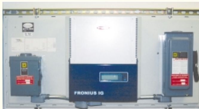
Fronius grid-tie inverter and optional AC & DC disconnect
