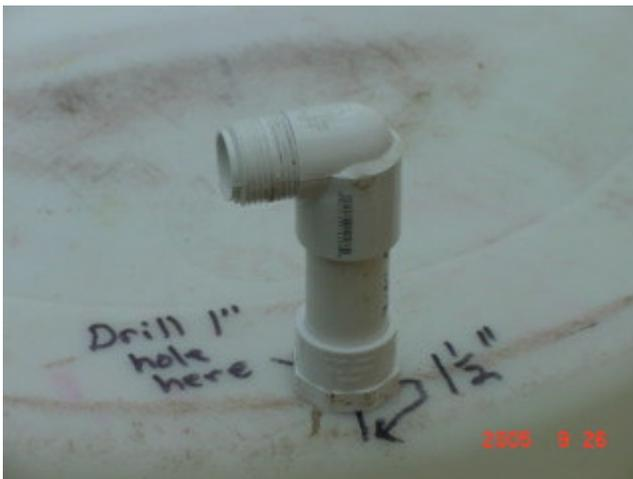
Install the ball valve and whatever fittings needed to hook up the pump you are using and the fish tank assembly is complete. It should look something like this.
