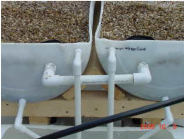
To prevent gravel from filling the balance tube use a short segment (usually about 6") of sewer pipe cut in half lengthwise at the mold seam. Remove the gravel in front of the balance tube fitting and slip one half of the split sewer pipe in front of the 1" pvc male adapter threads to create a void in front of the male fitting and backfill with gravel to hold in place. Do the same for the other side.
