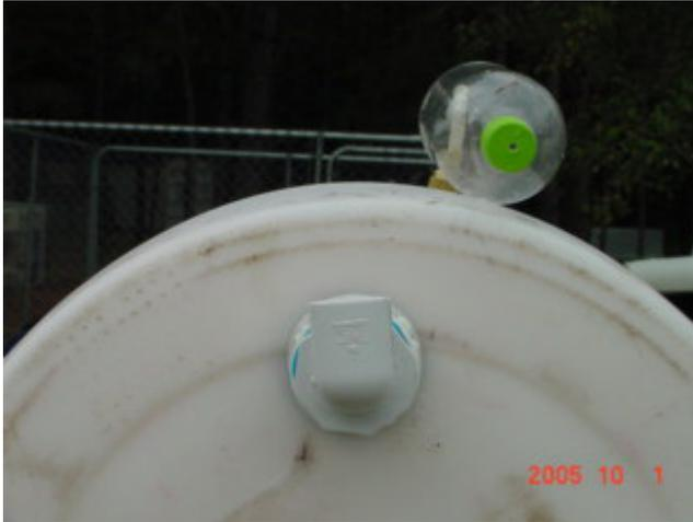
Sit the flood tank on the framework and install the manifold . The water bottle should hang to allow it to drain into one of the growbeds.
