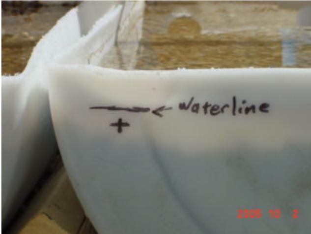
Install a 1/2" male pvc adapter into this hole with a 1/2" conduit locknut on the inside on each growbed. Insert a 4" long piece of 1/2" pvc pipe into the male adapter and install a 1/2" ell onto the pvc pipe and install a 12" piece of pvc pipe into each ell making a downspout for the growbed overflow protection. These should hang down into the fish tank as shown. Should any growbed siphon tubes get plugged the water will simply flow to the fish tank instead of on the floor.
