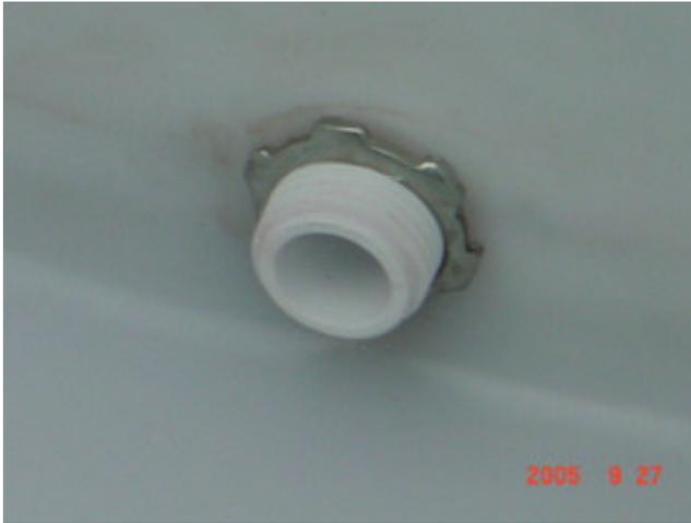
While holding the adapter with some pliers thread the 1/2" female x 1/2" barb to the threads protruding through on the inside. You have just made a bulkhead fitting with a 1/2" female pvc connection on the outside and a 1/2" hose barb on the inside. It should look like this.
