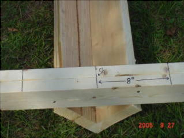
Screw 2 more 10' 2x4's together to form a 4x4 and cut into two pieces 51-1/2" long to form the longitudinal braces. Keep the excess pieces as they can be used in another part of the frame.
