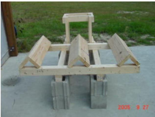
Set the barrel halves in the cradles as shown
