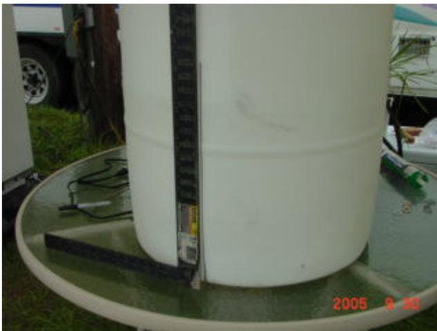
From the first vertical line make a mark at 9-3/4" from the bottom as shown and drill a 3/4" hole here.
