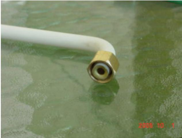
Assemble the to the fitting as shown and tighten 1/2 turn after the nut snugs up on the compression ring. This locks the compression ring to the pex pipe.
