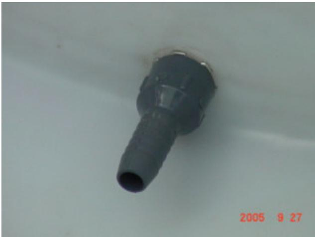
Slip the short section of hose onto the barb and ensure the curve of the hose is turned down.
