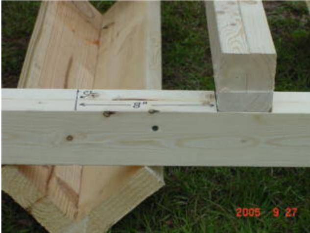
Screw these together using 3" deck screws as shown.
