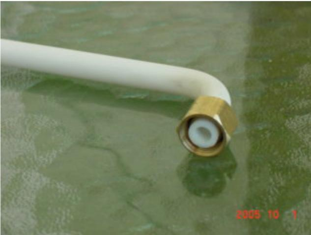
Take the inner tube slip it into the short end of the pex pipe.
