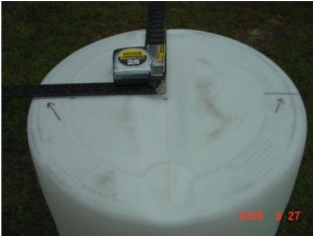
Be sure to make a mark on each side of the mold line and near the edge. This will be where the grow bed drains will be installed.
