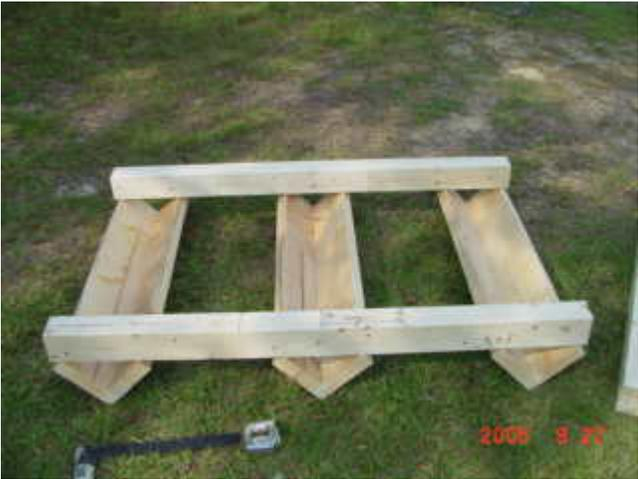
Mark the center of the cross brace as shown and measure out from there on each side 8".
