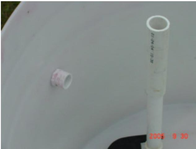
Install the siphon downspout from the outside as shown. Some sealer on the threads is helpful here. Tighten securely.
