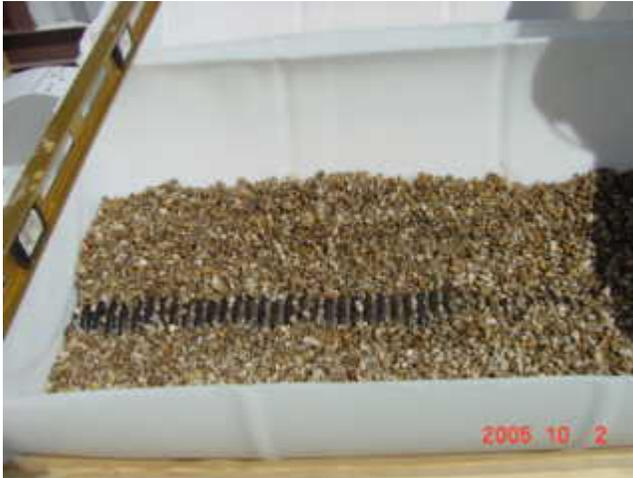
Finish filling the barrels with clean, washed pea gravel being careful to keep the tops of the barrel halves even and level. Fill to about 1" below the barrel bung holes.
