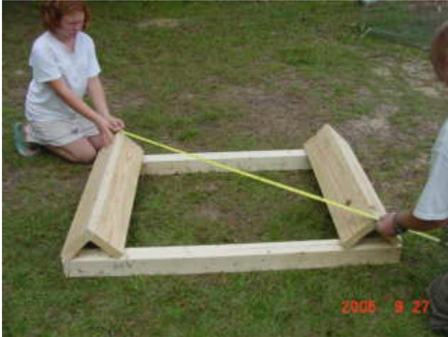
When they are equal screw the other four corners with 3" deck screws.
