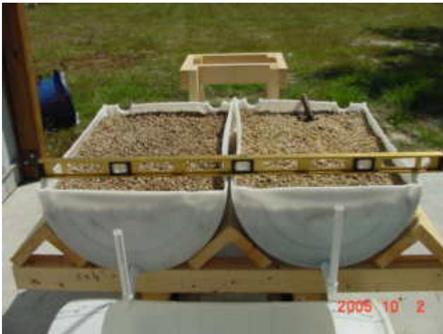
With a garden hose or some buckets fill the growbeds until the water level just comes up to the bottom of the barrel bung and mark the waterline on the front of the growbeds. Make a mark 1/2" below the water line and drill a 1/2" hole in each growbed at the location shown.
