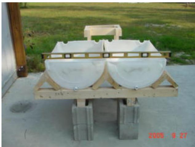
Position the fish tank and wedge it against the front blocks as shown with the remaining "V" piece.
