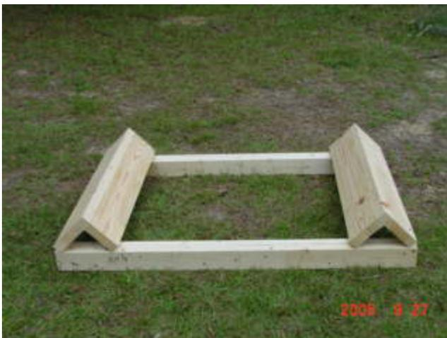
Put one 3" deck screw in each corner as shown and square the whole thing up by checking diagonals and moving until the diagonals are equal.
