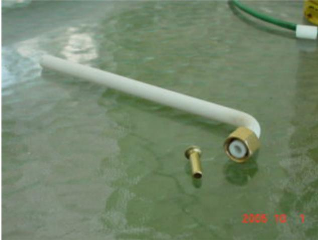
Reassemble the compression fitting finger tight for now and set aside.
