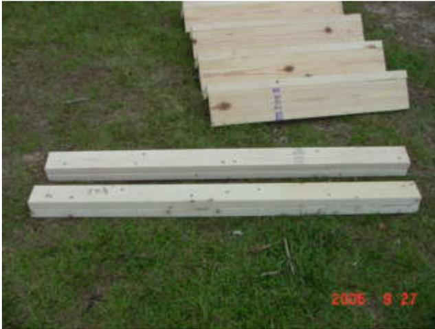
Next position these pieces on the ground roughly 36" apart and set the two of the "V" pieces on top to form a rectangle as shown.
