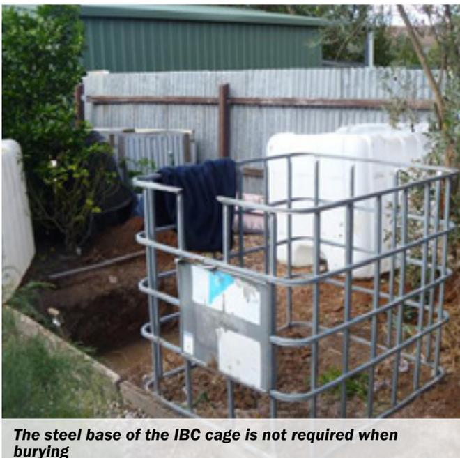
*The steel base of the IBC cage is not required when burying*
