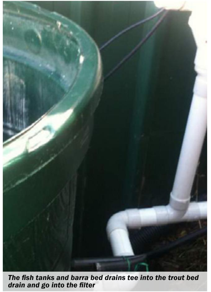
The fish tanks and barra bed drains tee into the trout bed drain and go into the filter
