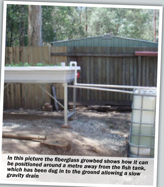
**In this picture the fiberglass growbed shows how it can be positioned around a metre away from the fish tank, which has been dug in to the ground allowing a slow gravity drain**
