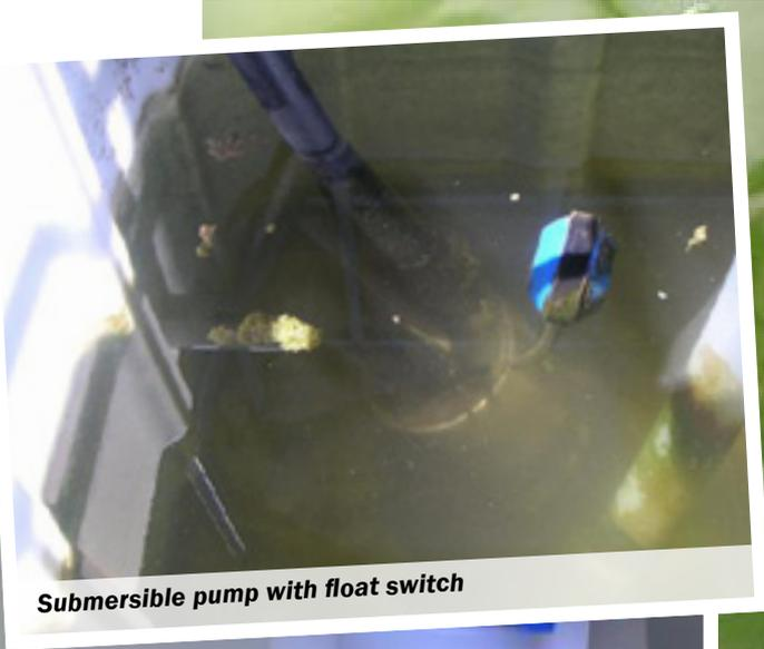
*Submersible pump with float switch*
