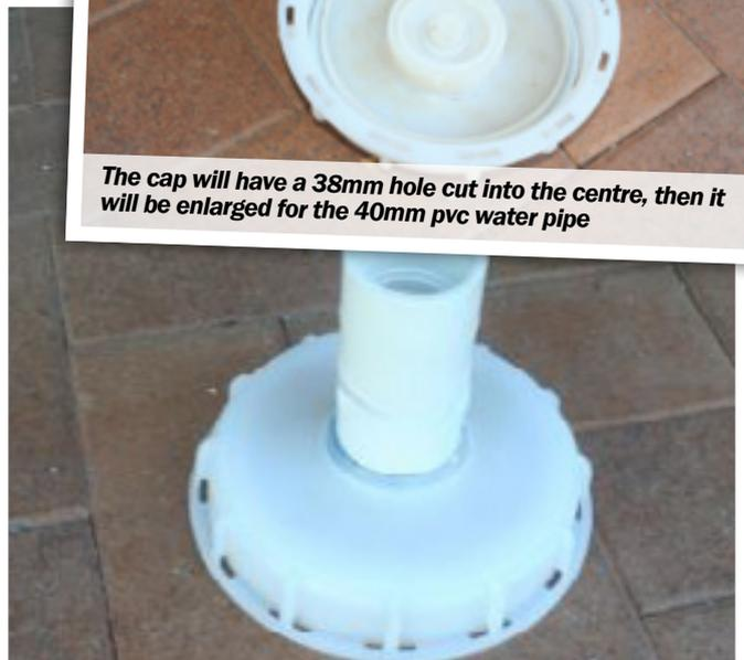
*Fittings installed in the lid of the IBC*
