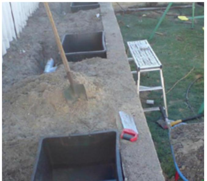
*The individual sumptanks for under each bed, buried and plumbed together*
