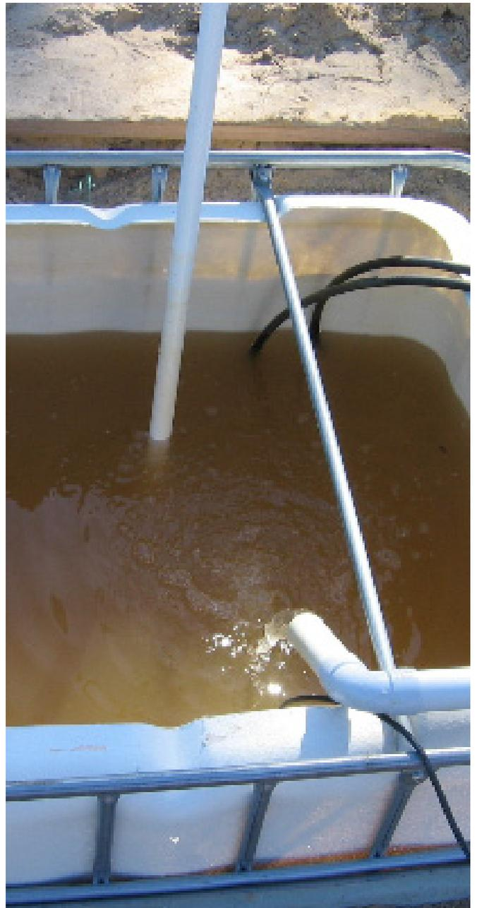
**Sump tank buried and supported in ground**
