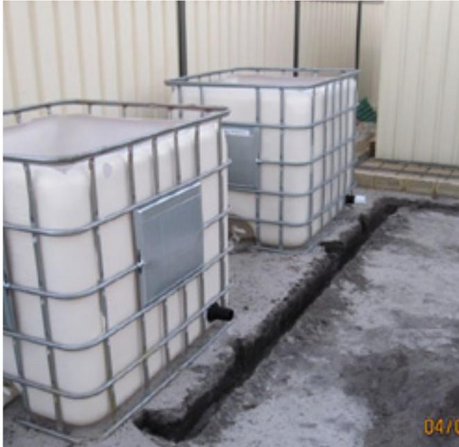
**1st 2 IBC's in place with tank fittings installed and trenches dug ready for pipe work**
