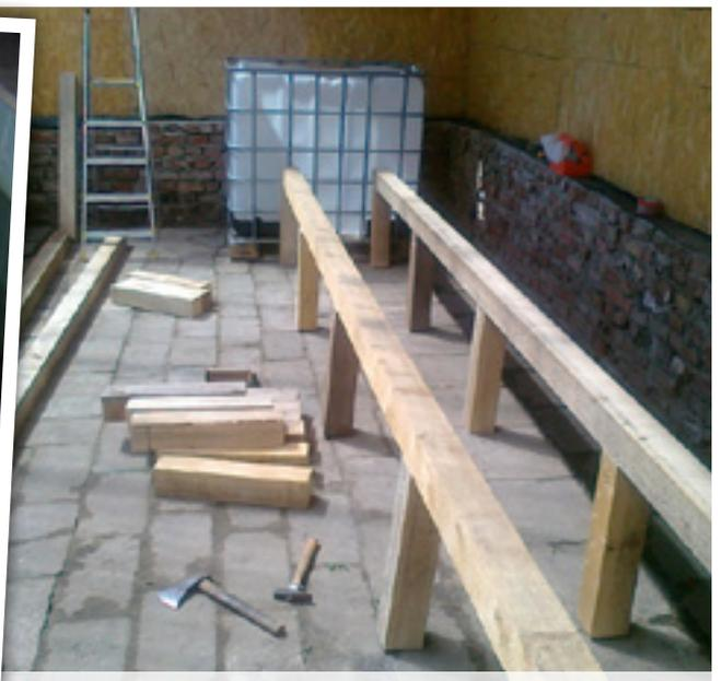
*Heavy duty beams to support the growbed*
