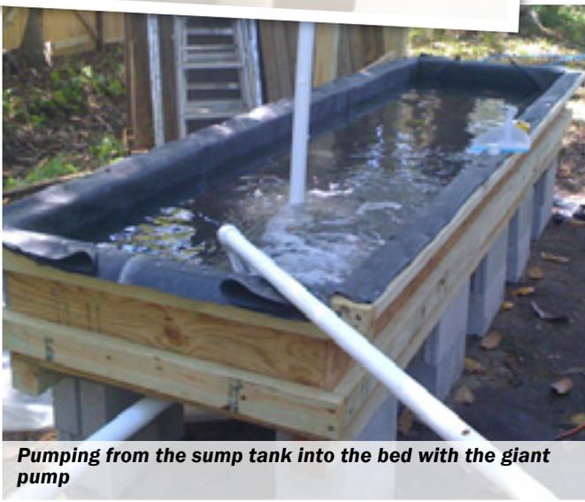
*Pumping from the sump tank into the bed with the giant pump*
