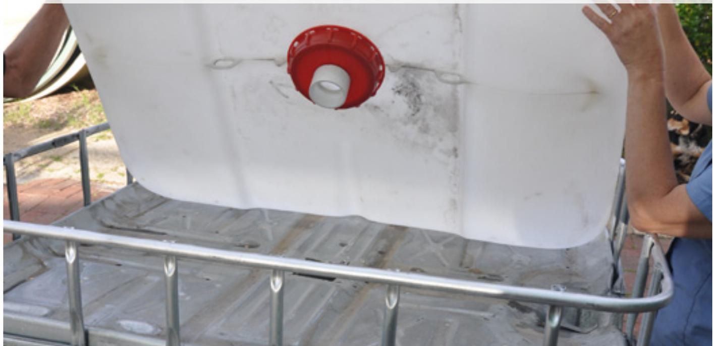
Now we place what was the upper section of IBC frame on the ground in the place where we want the system to be finally located. We then used two pieces of wood 30 x 50 timber from an old timber pallet to provide supports for the growbed frame. You can use a variety of different timbers for this purpose depending on what you have locally available in your area. You could just place the growbed onto the top of the metal frame, but by using timbers we
