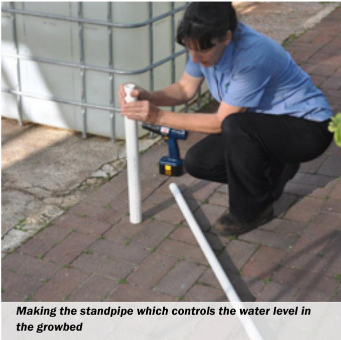
**Making the standpipe which controls the water level in the growbed**
