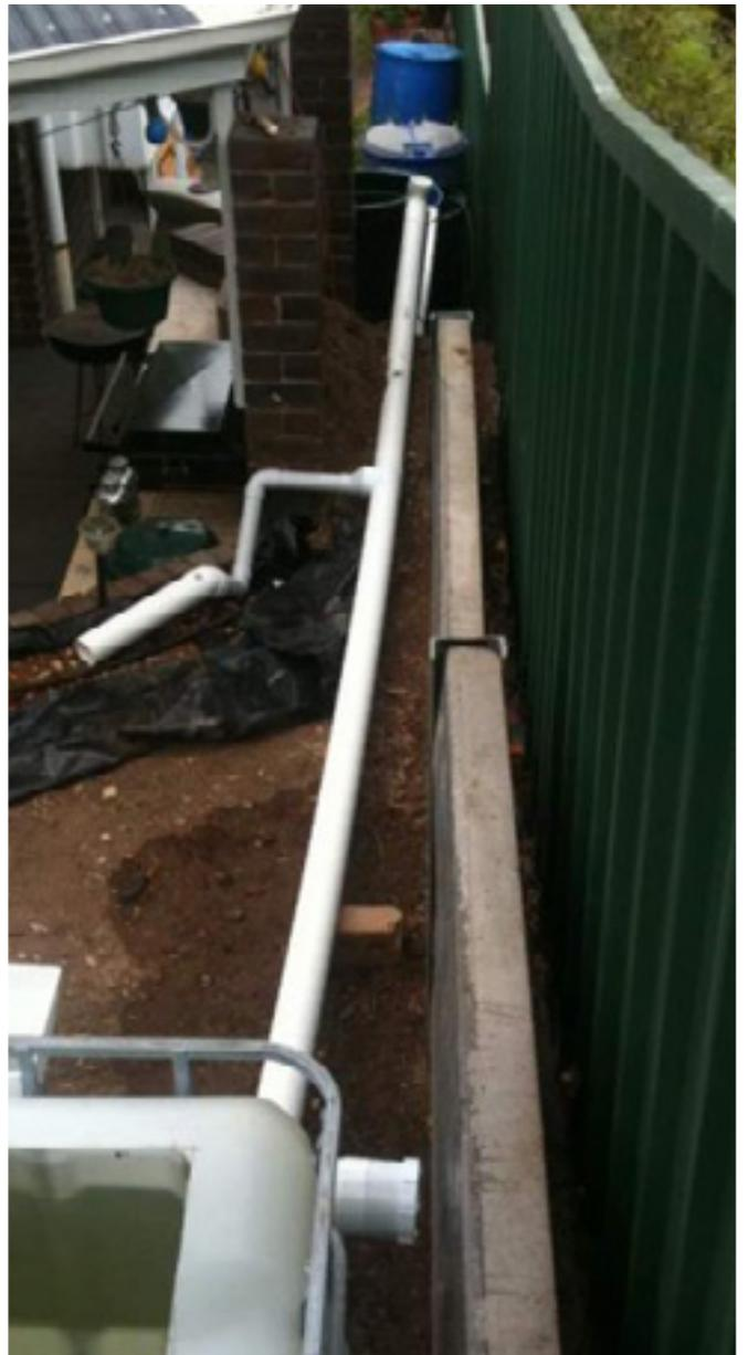
*Side view showing where they are situated in the backyard. Home made level control skimmer boxes. 90 mm storm water PVC with removable ends for cleaning*
