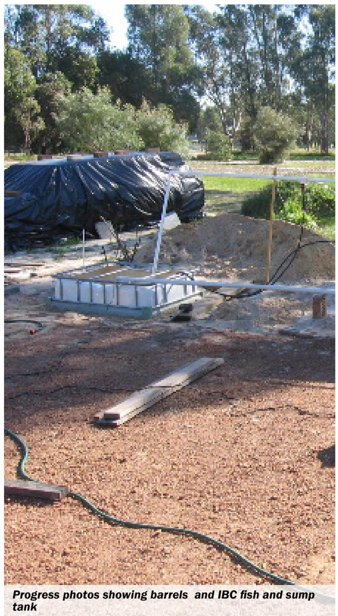
Progress photos showing barrels and IBC fish and sump tank
