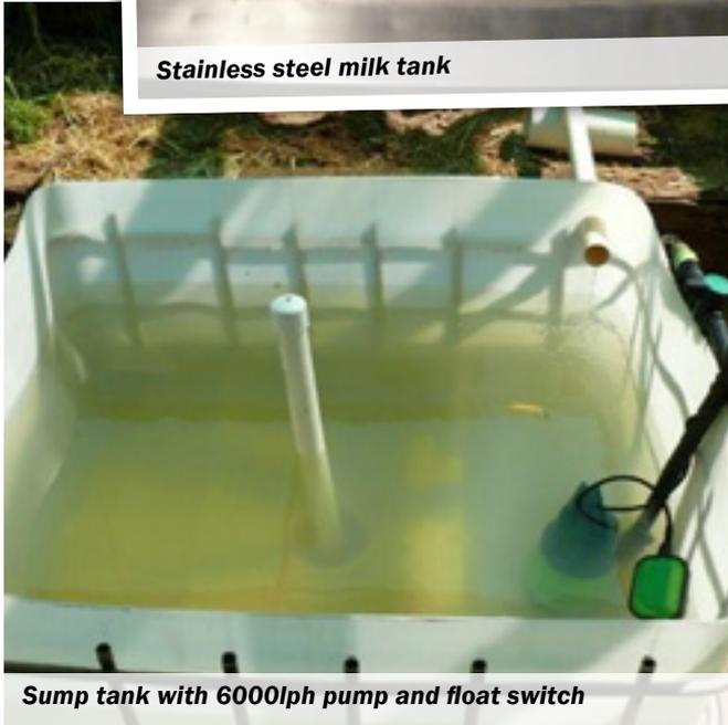
**Sump tank with 6000lph pump and float switch**
