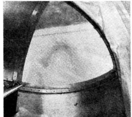
**PLASTIC FILM** is folded double under the clamps. Sheet-metal screws hold the two aluminum clamping strips. Plywood clamp at bottom is held by wood screws.
