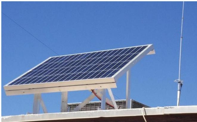
Straight South would have been better, but in order to tap into the roof beams for mounting it had to align with the orientation of the house. It still works great running lights, a fan (for the operator, not the
