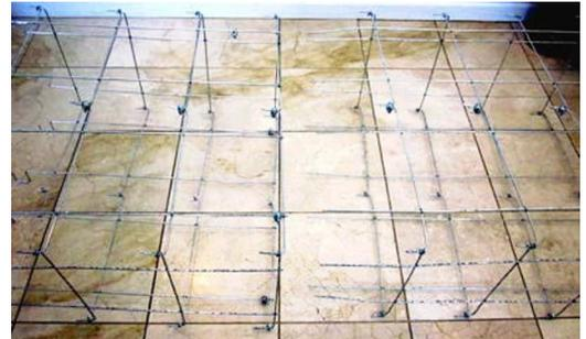
Be sure to feed the all of the legs of the extension cage **outside** the base cage. When clamping the Clips down, keep the overlap to a minimum as this directly affects the final cage height.
