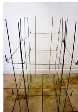
**Step 9:** Place Wire Rope Clips on the 4 vertical rails on the outer top sides of the base cage. (These will loosely sit on the 4 vertical legs at the top rung for the moment. They will be slid to the top of the rails for anchoring the extension cage.)
