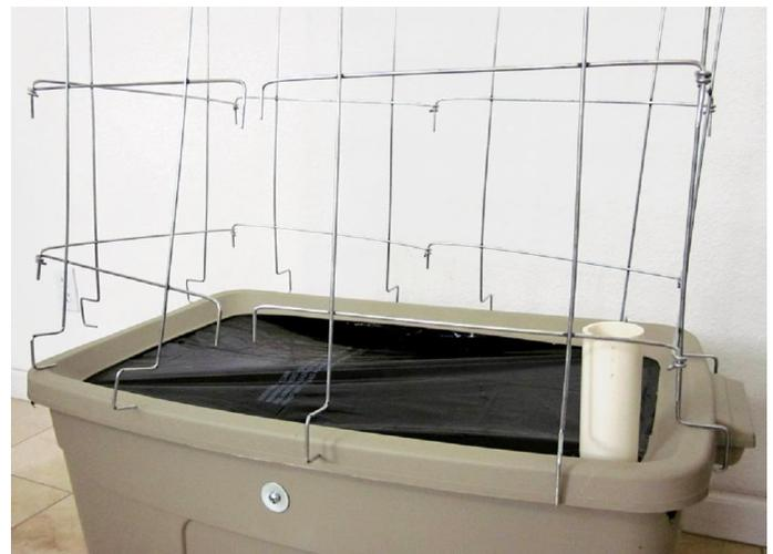
With a person on the back-side and another one on the front-side, continue working the cage legs from right to left around and under the rim.
